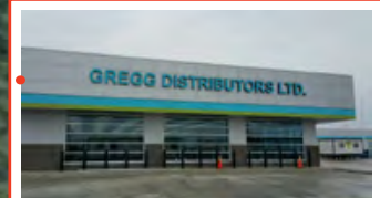
Gregg Distributors 7180 Boundary Rd 70,000 Sf Logistics Facility
